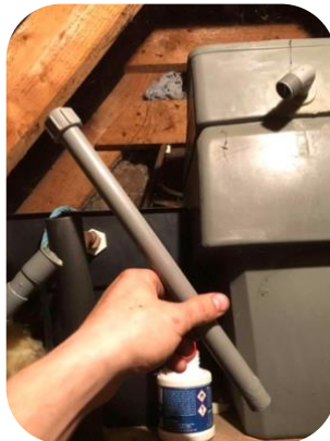
The overflow pipe being installed
