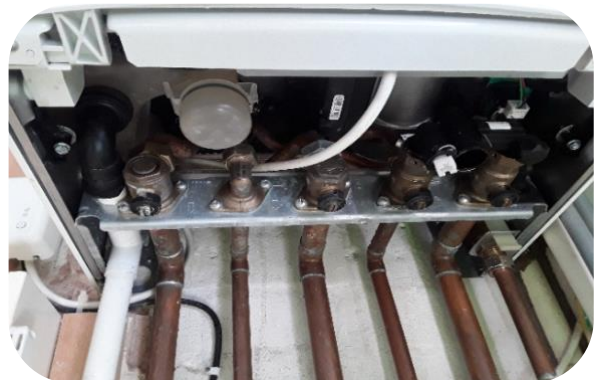
New boiler condensing trap installed
