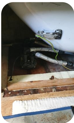
New flexi hose & earth bonding installed
