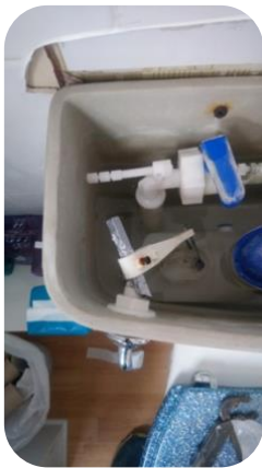
Damaged toilet handle
