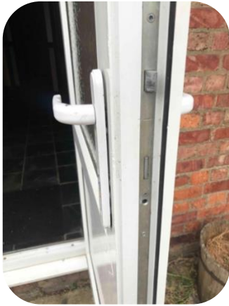
Damaged PVC door lock
