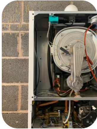
Old expansion vessel removed
