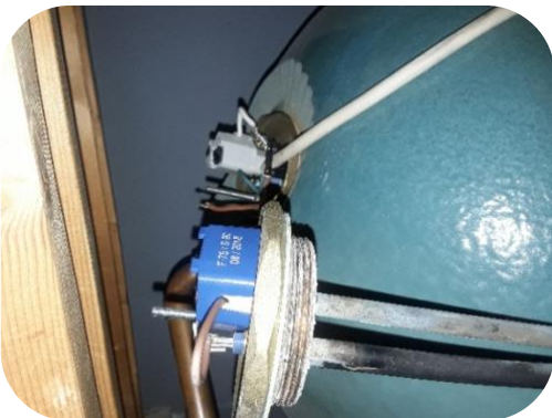
Old element being removed
