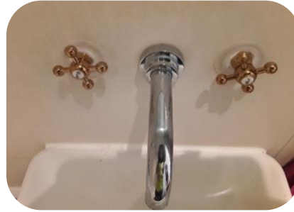
New mixer taps installed
