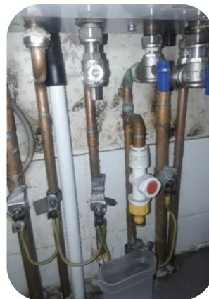
Installed new compression boiler valves
