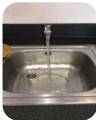
Installed new sink & mixer tap
