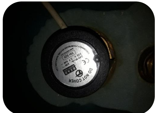
New cylinder heating element installed
