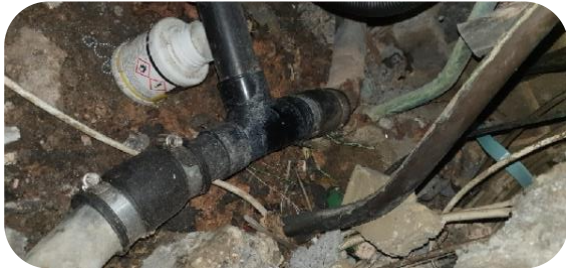
Repair to leaking joints under bath
