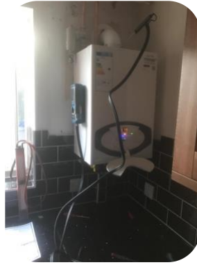
New boiler being commissioned
