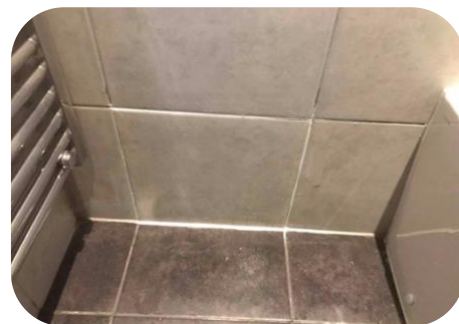
New grouts on tiles
