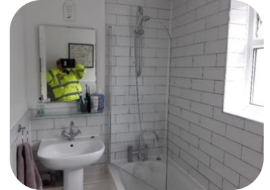
New bath screen installed
