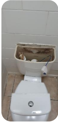
Replacing toilet flusher
