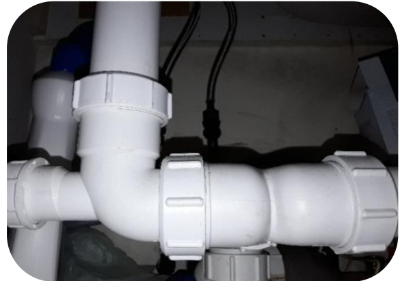
New trap installed
