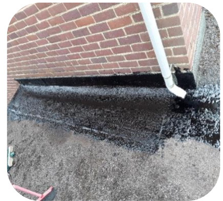
Repaired roof & reapplied roof tar
