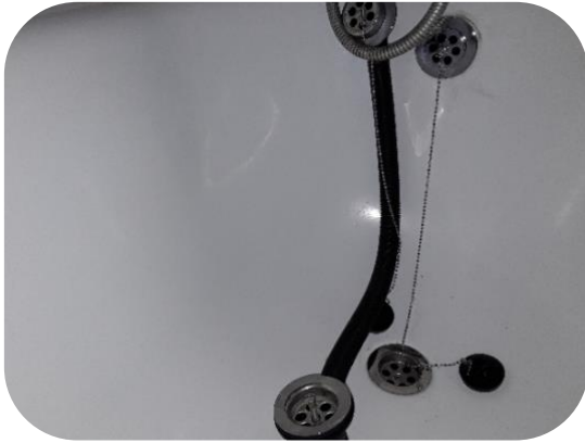
Replacing bath overflow waste pip
