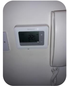
New room stat installed
