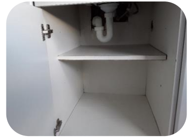
New under sink waste trap installed
