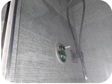
Old cartridge removed
