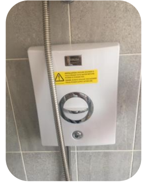
New electrical shower installed
