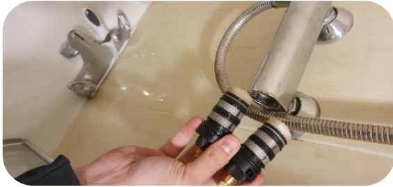
Replacing shower valves
