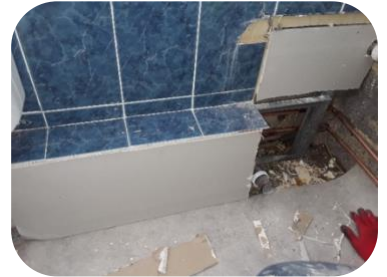
Replacing pipework inside boxing
