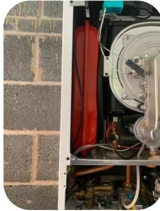
New expansion vessel installed
