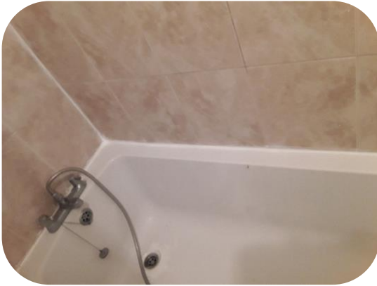
Applied silicon around bathtub
