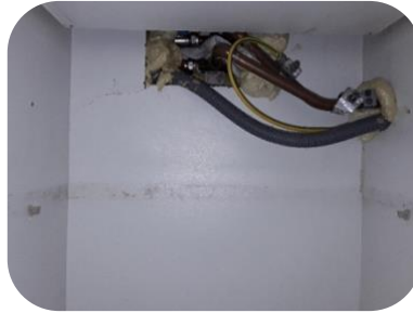
New earth bonding & WM inlet hose
