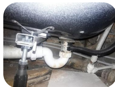
New trap installed under bathtub
