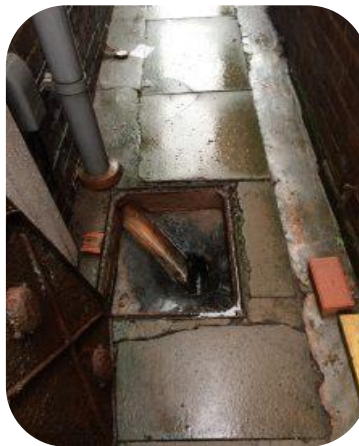
Unblocked manhole & tested water running
