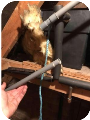
Old snapped overflow pipe
