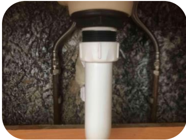
New waste pipe installed
