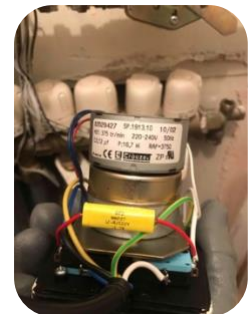
New pump motor installed
