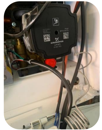
New pump fitted
