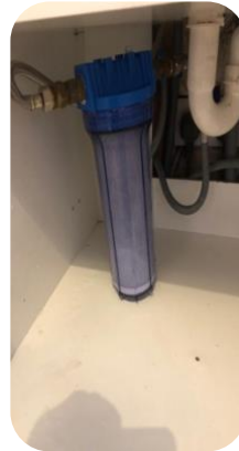
New water filter installed
