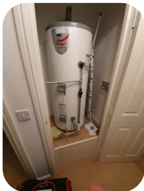
New vented MEGAFLO cylinder installed
