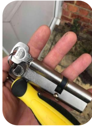
Installed new PVC door lock
