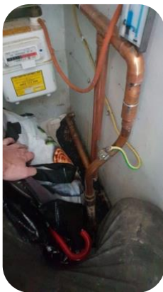
Upgrade gas meter outlet pipework from 15mm to 22mm
