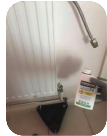
Chemicals added to central heating system
