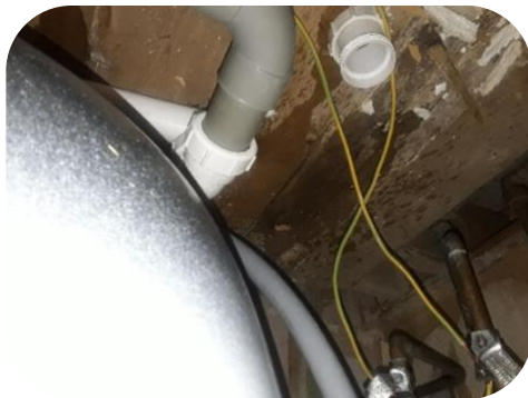
Installed bathtub waste pipes
