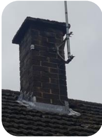
Chimney pointed & new lead flashing
