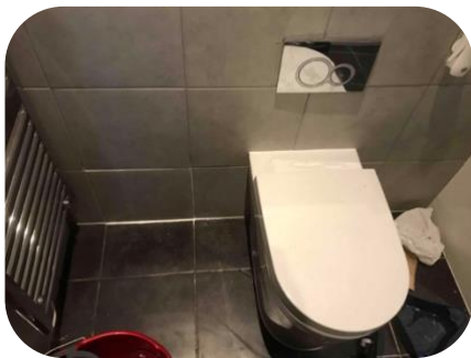
New toilet installation
