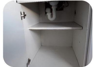
New under sink waste trap installed
