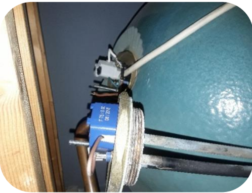
Old element being removed
