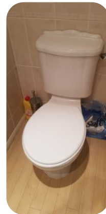
Supplied & installed new toilet & lino flooring
