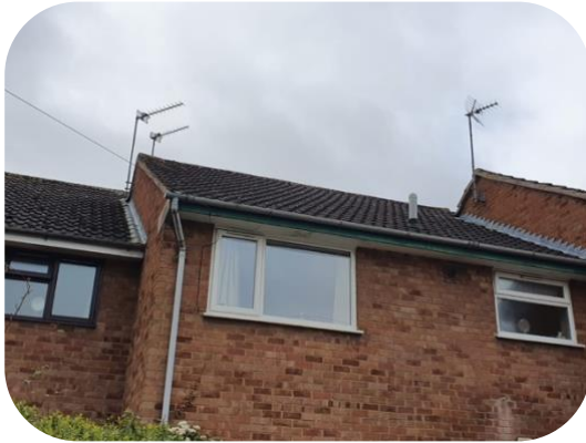
Installation of new gutters
