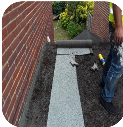
During roof work
