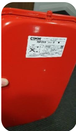
Installation of a new expansion vessel
