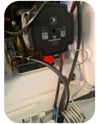
New pump fitted
