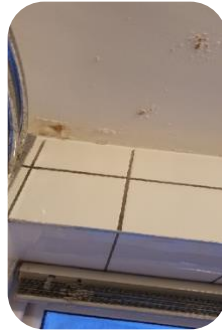
New tiles installed
