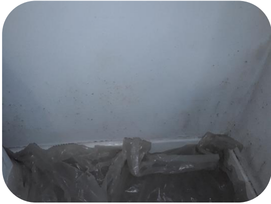
Dust sheet installed before painting
