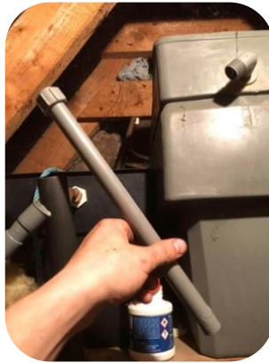
The overflow pipe being installed
