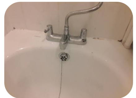
New mixer tap installed
