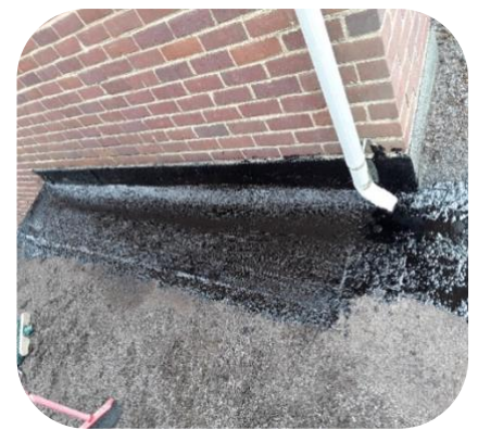
Repaired roof & reapplied roof tar
