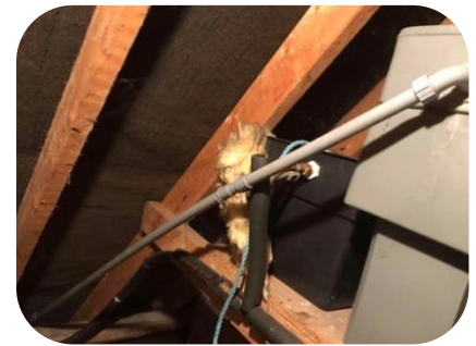
New cold-water tank overflow pipe installed
