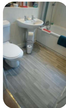
Installation of vinyl floor (after)
