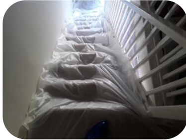
Covering carpets to prevent damage
