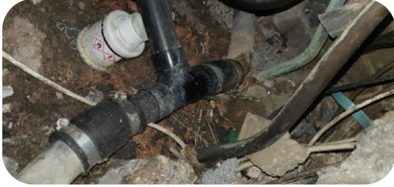
Repair to leaking joints under bath
