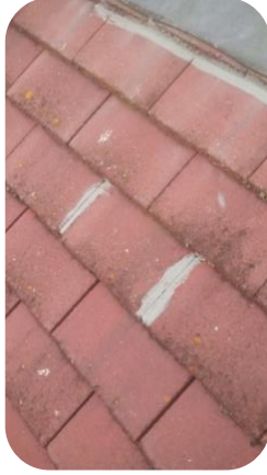
Damaged tiles replaced
