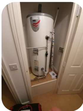
New vented MEGAFLO cylinder installed
