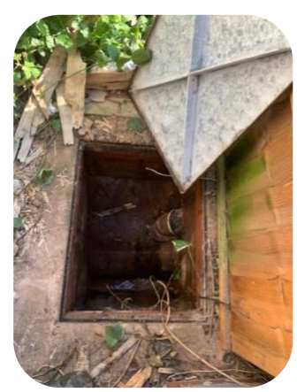
Inspected all the manholes around the property
