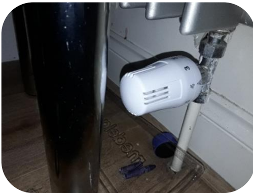
Installed new PRV valve
