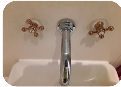
New mixer taps installed
