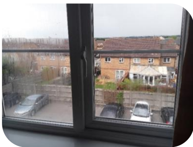
Adjusted & repaired the PVC window
