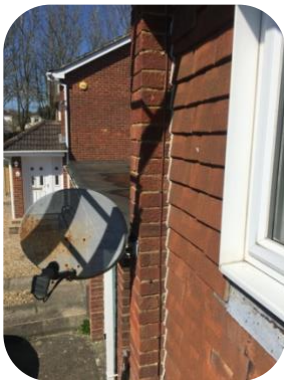
Repair to TV aerial
