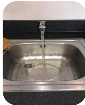
Installed new sink & mixer tap
