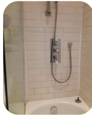
New tiles installed, grouted & made good
