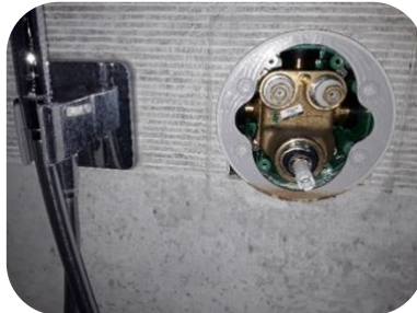
Installed new cartridge
