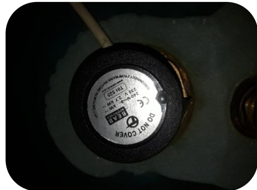
New cylinder heating element installed
