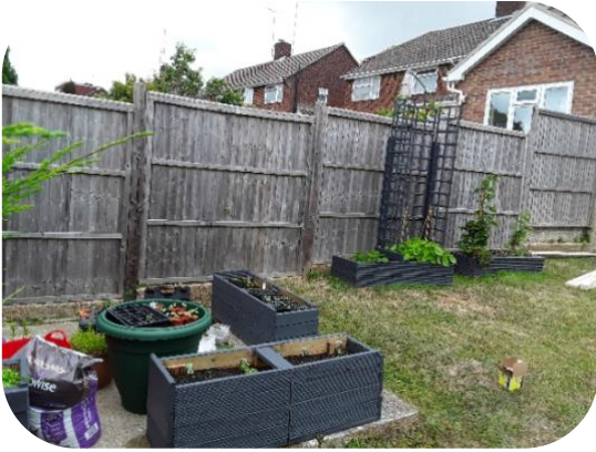
New fence installed
