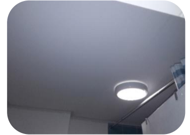
New ceiling installed
