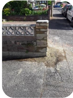
Repaired entrance wall
