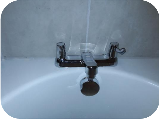
Installed new bath mixer taps
