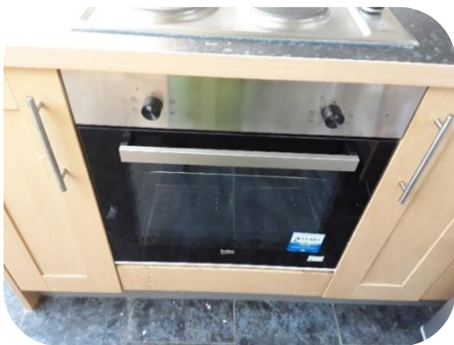
Supplied & installed new oven
