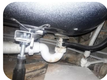
New trap installed under bathtub
