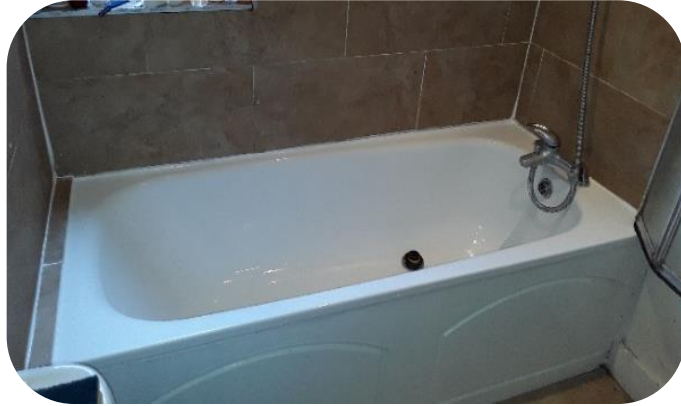
New bathtub & new tiles installed
