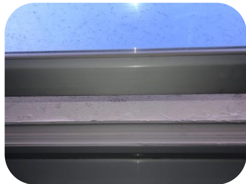
Installed new window rubber and window hinge
