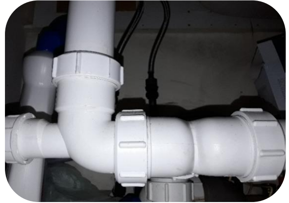
New trap installed
