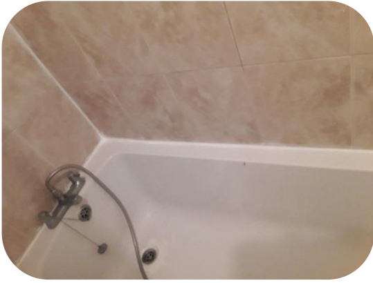
Applied silicon around bathtub
