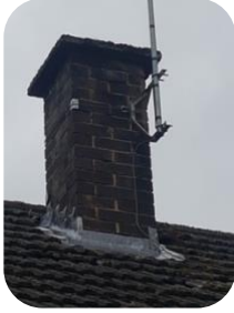
Chimney pointed & new lead flashing
