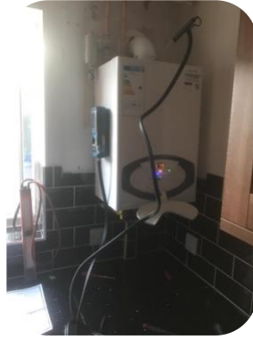
New boiler being commissioned
