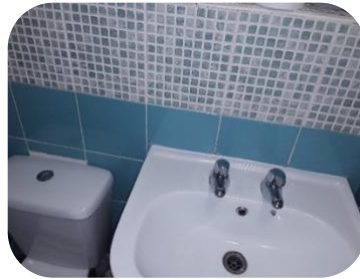
New sink & toilet installed
