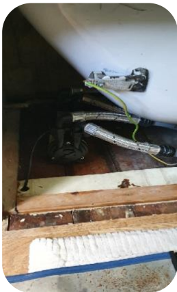
New flexi hose & earth bonding installed
