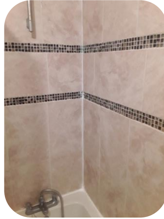
Grouted all bathroom tiles
