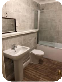
New bathroom, tiling & flooring installed
