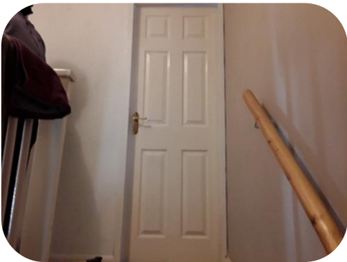
New fire door installed
