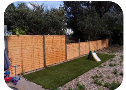
Garden left clean after fence installed
