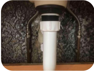
New waste pipe installed
