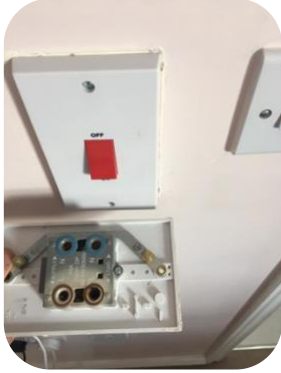
Isolation switch replaced
