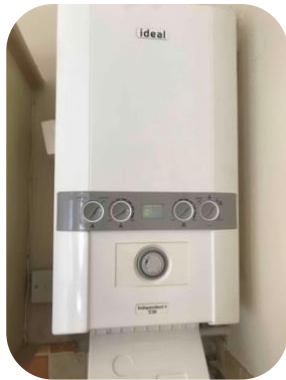
Installed new Ideal boiler
