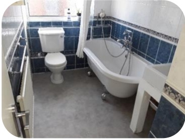
New bathtub toilet & sink installed
