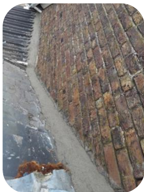
Sealed full roof hips
