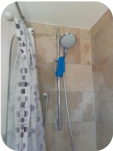
New shower handle railing installed
