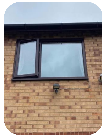
Installed new window
