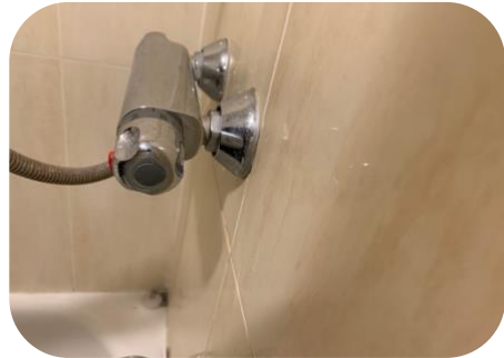
Tidy job, tiles were not damaged
