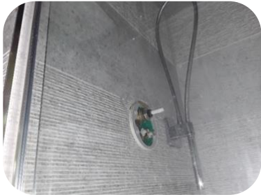
Old cartridge removed
