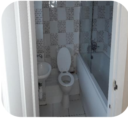
Installed new Full Bathroom
