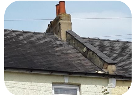
Full repointing of the roof
