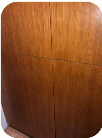
Adjusted & repaired fallen wardrobe
