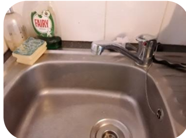
New mixer taps installed
