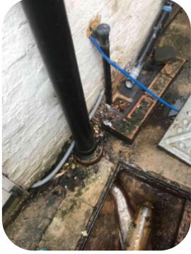
Cleaning drains following removal waste
