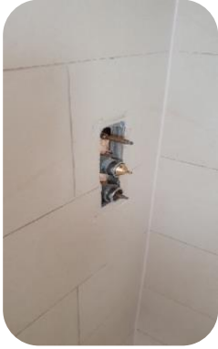
Installation of new shower cartridge
