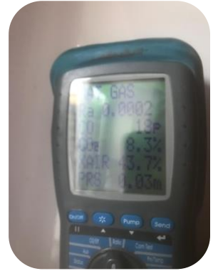
Flue test on new boiler
