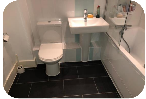
Pipework boxing (after)
