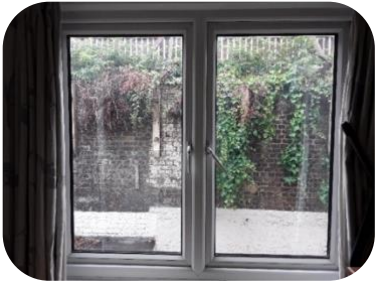
New PVC window installed
