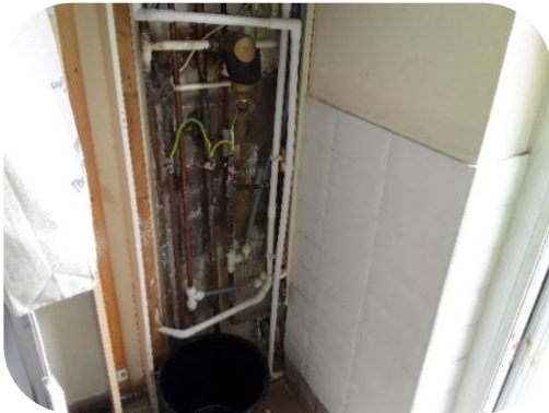
Installed new condensing pipe
