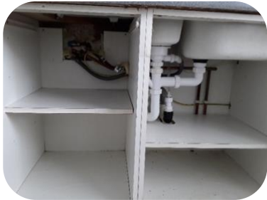
New sink trap & waste connectors
