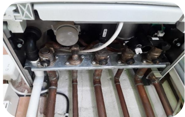
New boiler condensing trap installed
