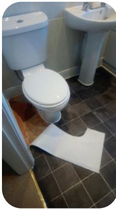
Installation of vinyl floor (before)
