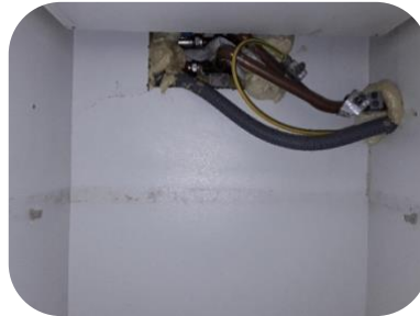
New earth bonding & WM inlet hose
