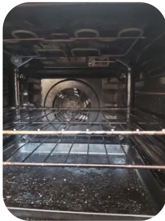
New oven fan & heating element installed
