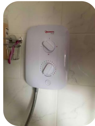
Installed a new shower
