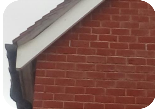
New lead flashing installed
