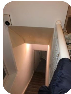
Installed new bannister
