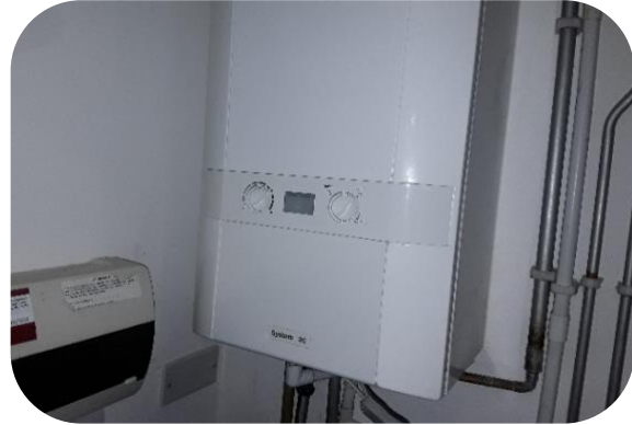
Installed new boiler
