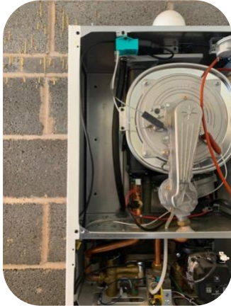
Old expansion vessel removed
