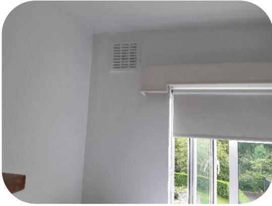
Painted living room after repairs to walls
