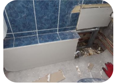
Replacing pipework inside boxing
