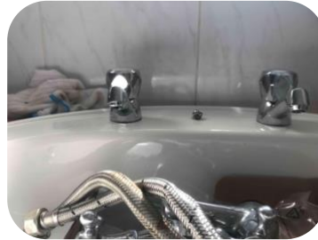
New mixer taps following replacement
