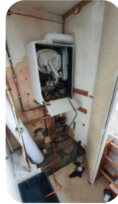
Testing boiler for safety following the work
