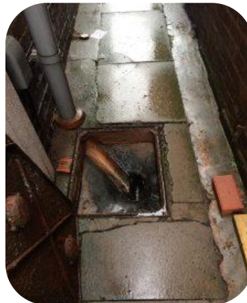
Unblocked manhole & tested water running
