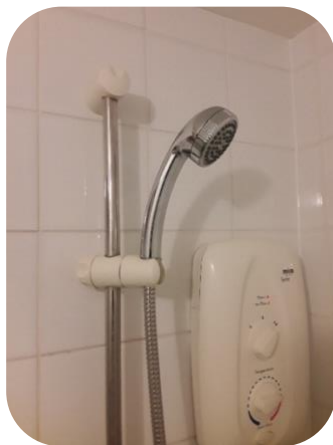
New shower installed
