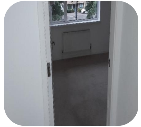
Installed new carpet & new PVC window
