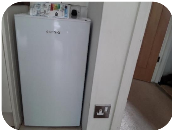
Installed 50cm wide fridge, with new power point
