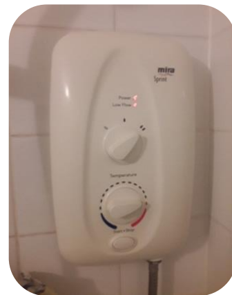
New shower tested working
