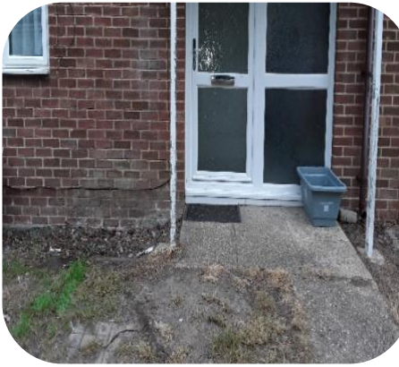
Installed new PVC Entrance door
