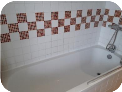
Installed new bath, tiling and sealed
