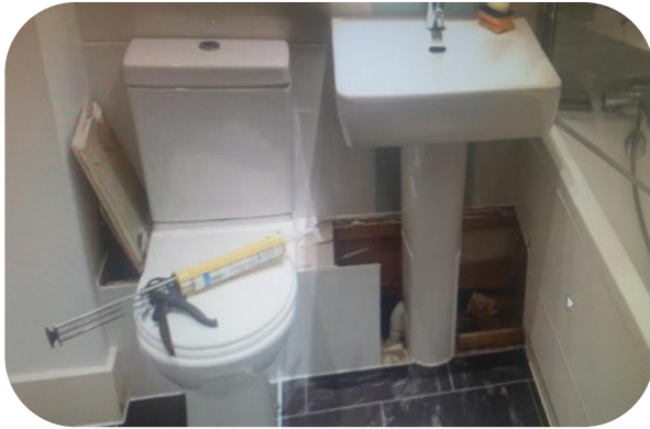
Pipework boxing (before)
