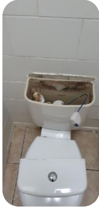
Replacing toilet flusher
