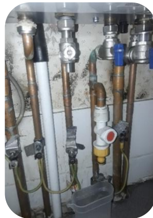
Installed new compression boiler valves
