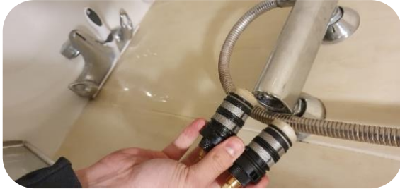
Replacing shower valves
